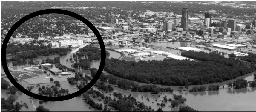
Figure 5: Water Works and the 1993 Flood 56
